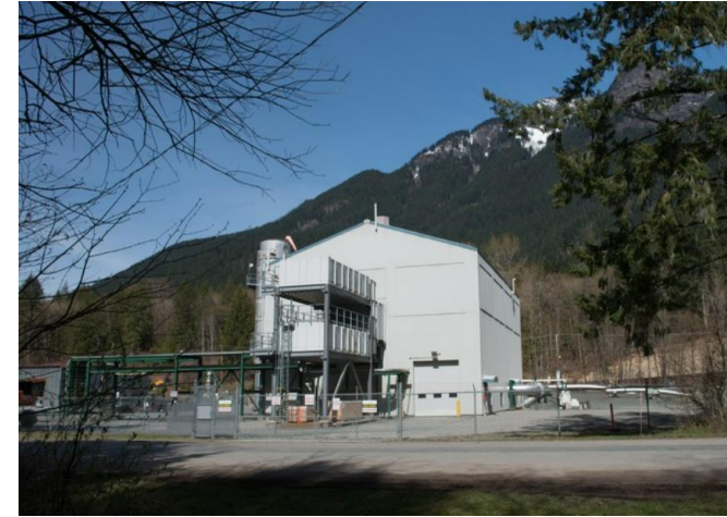
Compressor station "8B"
