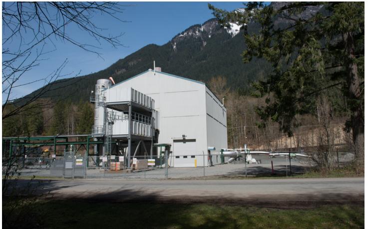
> Compressor Station 8B (CS-8B “Othello”)
