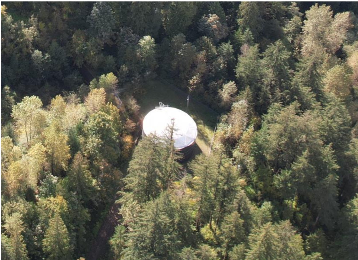
Photo 4. Critical Infrastructure: water reservoir in the wildland-urban interface.
