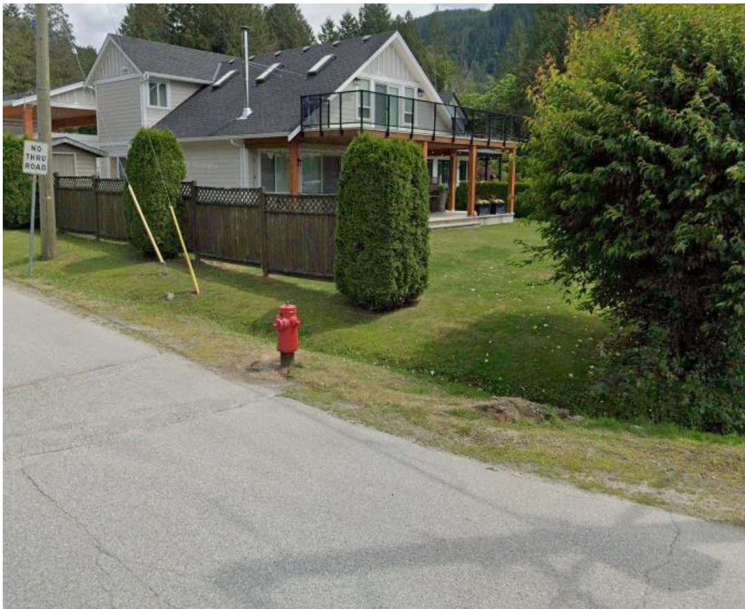
Photo 5. Hydrants in the Kawkawa Zone may not provide sufficient water supply for fire suppression.
